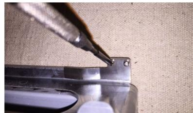
10. Remove the backgage sensor upper and lower brackets.
